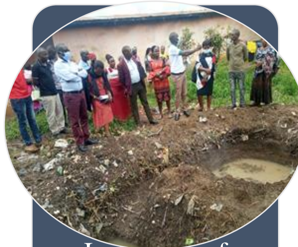
Inspection of excavated pit to sediment grey effluent before discharge in to Mpanga behind Mpanga market – Fort Portal City
