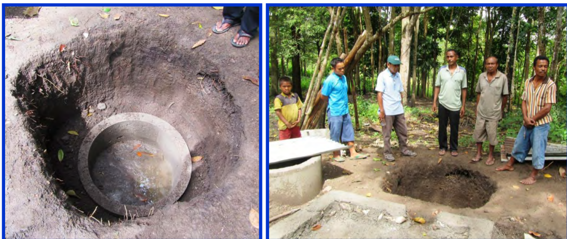
Pour-flush toilet under construction in Plan Indonesia STBM village (Sapaen village)
