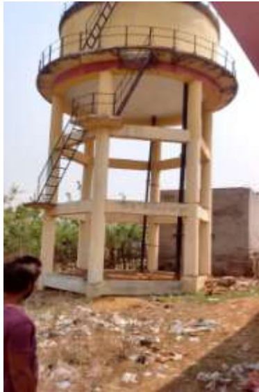
Pic 6: A dysfunctional government overhead tank in Kanamana, Ganjam
