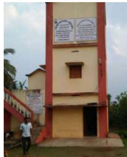
Pic 7: Overhead tank built & maintained by Gram Vikas in Kanamana, Ganjam
