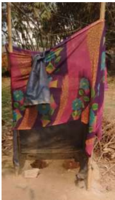
Pic 17: Self built pit toilet. Woman in rural Samastipur uses it and covers the faecal matter daily with ash from her wood fire cook stove.
