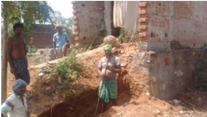
Pic 14: Note the elevated foundation to prevent flooding.
