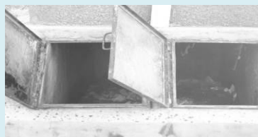
Two chamber and vaults of ECOSAN used at the same time by teachers in Alune P/S, Akwang Sub County
