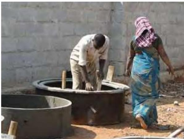
Production of rings of holding tank
