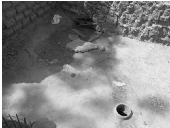
Figure 2.20 A typical traditional latrine in Mali. Note the circular rim of a clay pot used to line the latrine hole. The rock slab near the drainage hole in the upper part of the photo is the area typically used for bathing. Use of latrines and bathing areas pose special physical and hygienic challenges for disabled persons, especially if the floor is muddy, poorly drained or unkempt by the rest of the household.
