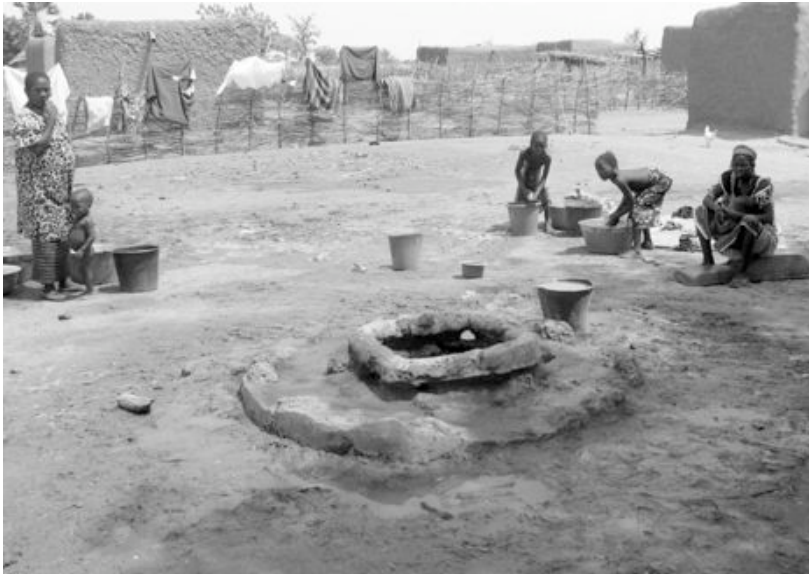
Figure 2.6 Traditional village well in south-central Mali. Note the poorly constructed apron and the standing water and mud surrounding the well.
