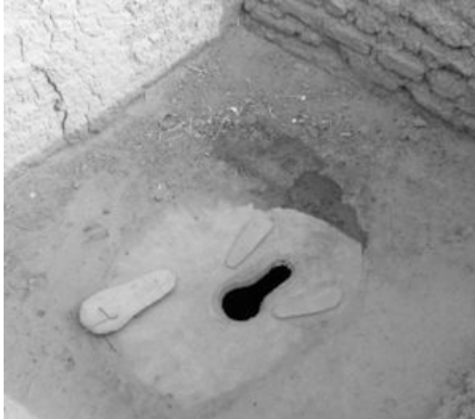
Figure 6.3 A sanplat latrine soiled by urine from improper use and poor drainage.
