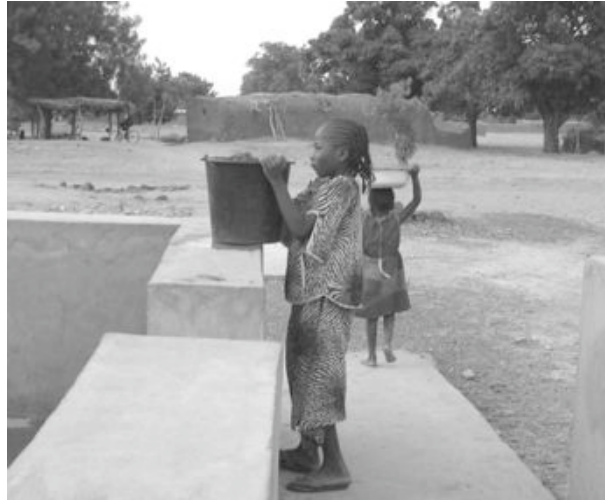
Figure 4.10 By separating the lifting motion into two less strenuous steps, lower enclosure walls can be used to facilitate lifting heavy water containers to the head for transport (i.e., lifting from floor to wall, then from wall to head).
