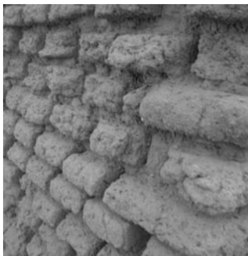
Figure 6.8 Exposed clay brick walls in the interior of latrines, while subject to deterioration by seasonal rains, can provide helpful handholds and support for some disabled and elderly persons.
