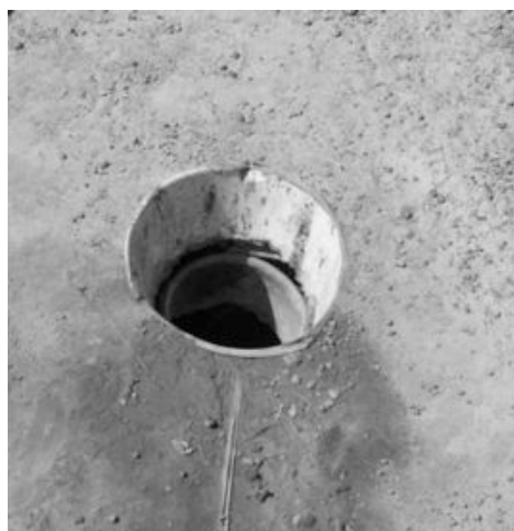
Figure 6.5 A traditional latrine used by a disabled person who, due to lack of adequate leg strength, must sit directly on the hole. Note the rim of the hole (the remains of an old metal container) is flush with the ground surface so as to minimize discomfort when the user is seated on the ground.
