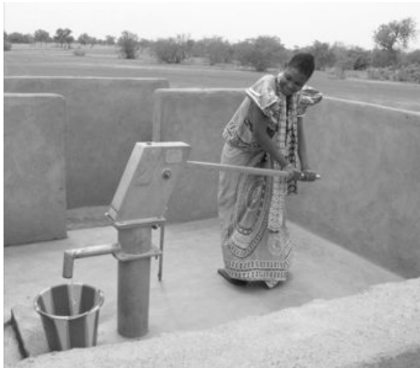
Figure 4.2 This young mother and polio victim can only walk with the aid of crutches, but she uses the pump handle to steady herself, freeing her hands for pumping. She is unable, however, to produce a steady pump flow because much of her strength is used to stabilize herself, leaving little strength for stroking the pump handle.
