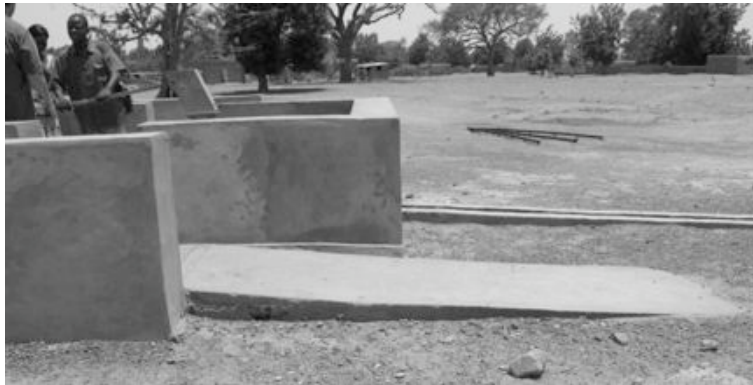
Figure 4.7 Side view of a pump superstructure access ramp.
