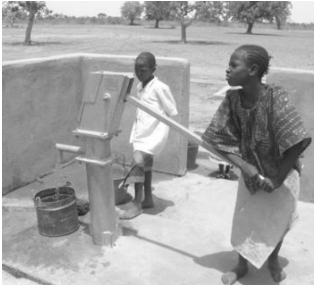
Figure 1.4 A typical hand-pump and superstructure facility of the Mali Rural Water Project
