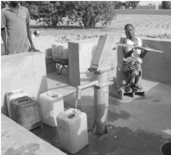
Figure 4.19 A disabled woman assists with preliminary testing of side-seat positioning.
