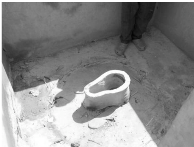
Figure 6.16 Terra cotta latrine seat in use on a sanplat latrine in the home of a polio victim. When not in use, the seat is moved to the side of the enclosure for storage.
