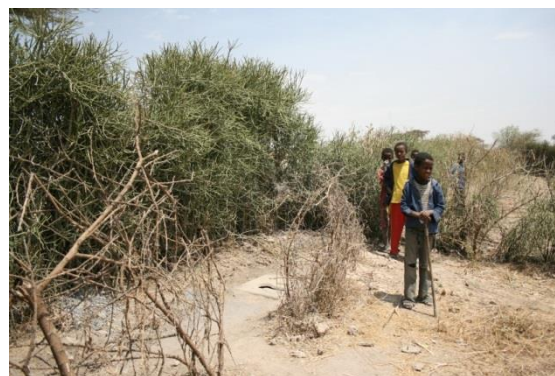
Figure 2. Arborloo without superstructure, East Arsi (March 2013).
