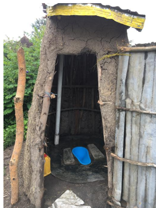
Figure 2: Respondent's SATO pan toilet installed on a concrete slab
