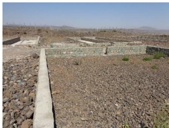
Photo: A completed Sludge Drying Bed in Welenchiti town, Oromia Region. (Photo by UNICEF, May 2017)
