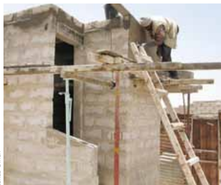
Photo 1: Construction of a dehydration toilet in Nouakchott.
