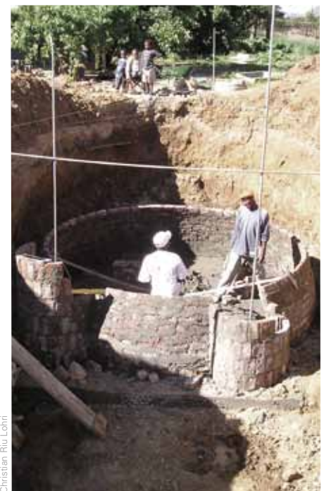
Photo: Construction of a fixed-dome underground biogas digester in Lesotho.
