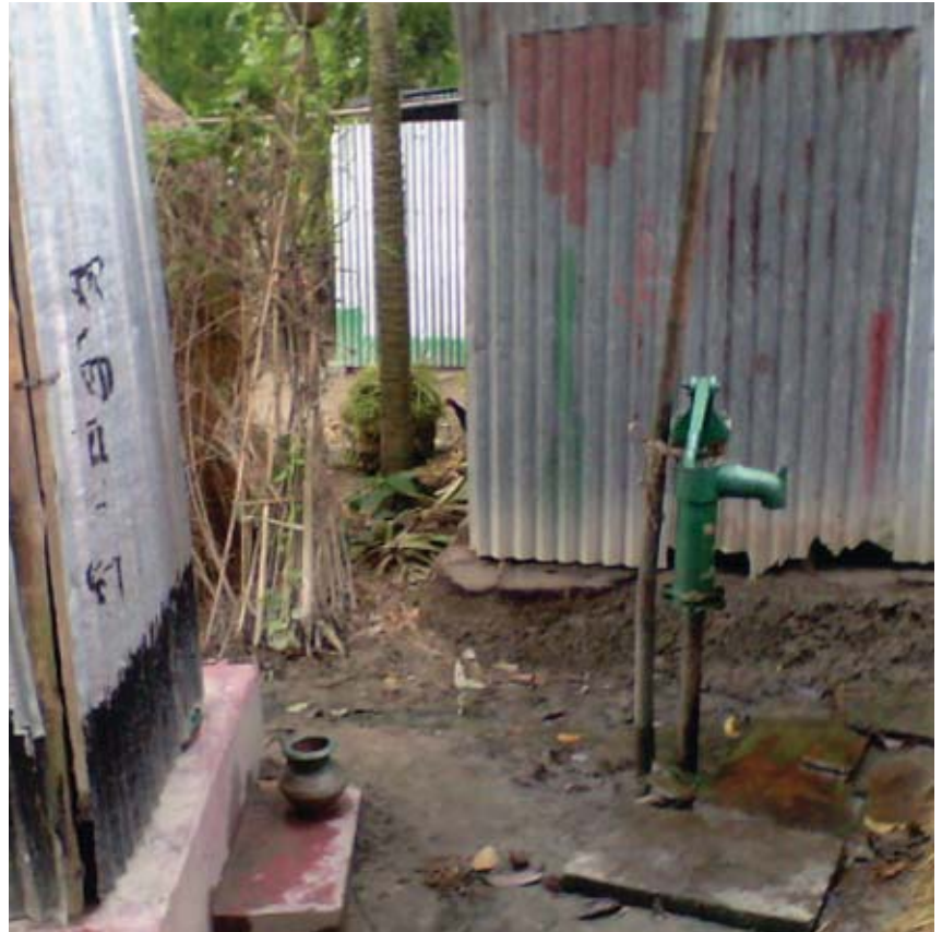
One issue that the M&QC team examines is whether latrines are constructed too close to water points so that they might compromise water safety.
