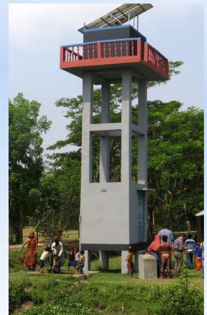
Low-cost, community-scale piped water system with water tower (implemented by GIZ) in Samnashi, Bangladesh. Note the solar panel on the top of the tower. © Ebo Roek
