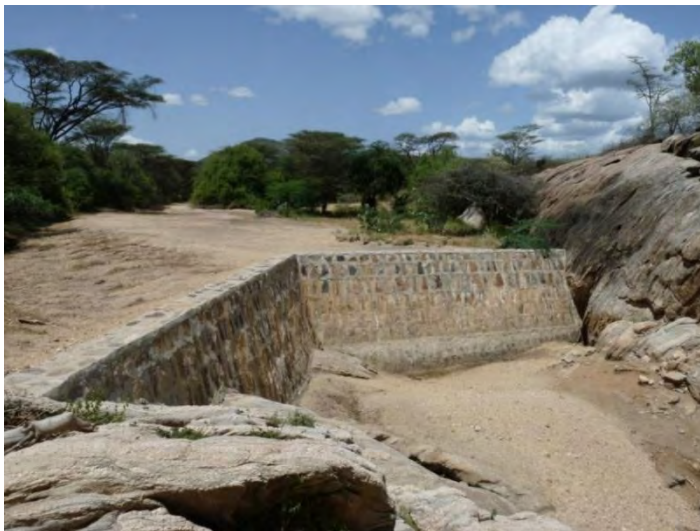
Figure 2 Sanddam near Nakabosan, Turkana
