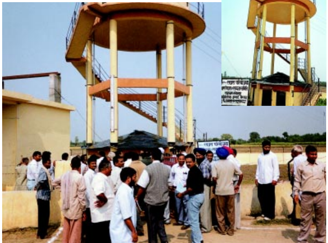
Participants on a study tour observing how villages constructed, and now operate, their own water supply.
