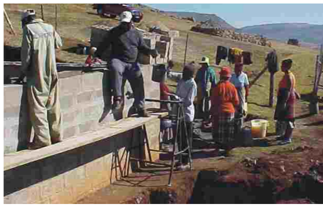
Building the reservoir
