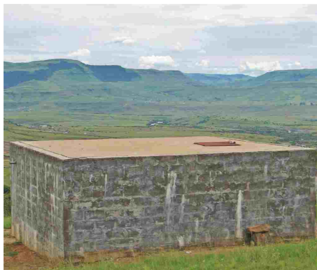
Finished reservoir in operation
