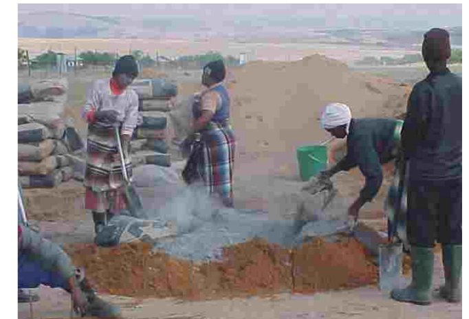
Manufacturing cement blocks for reservoir and pumphouse walls
