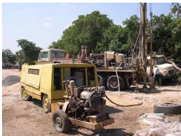
Figure 2 – Large rig mounted on a truck
