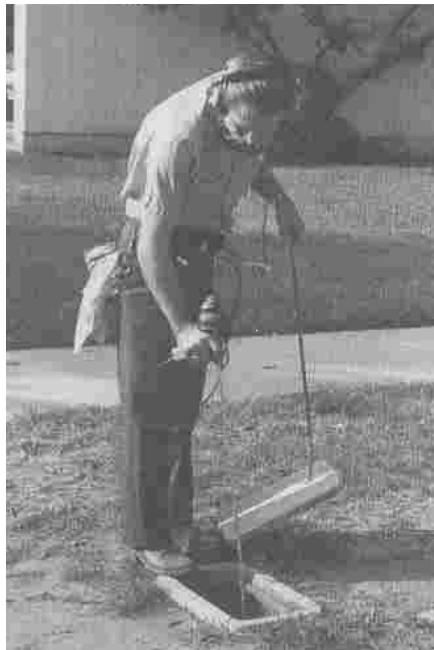
Figure 8-3 Listening for leak noise at meter
