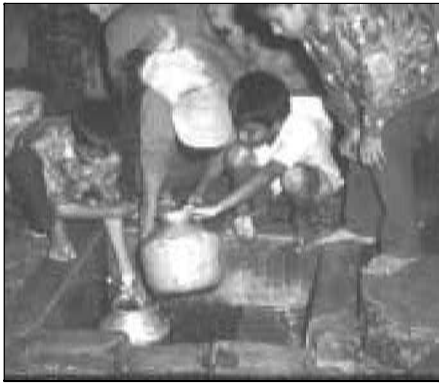
Pressures are often so low that outlets often have to be below ground-level
