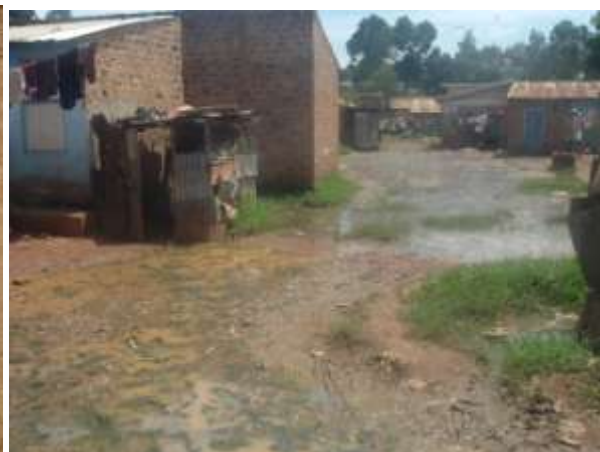
Picture 2: Flooded waste water during rain season
