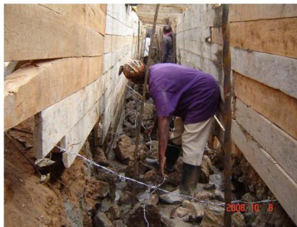
*Figure 3. Artisan in trench showing form work, steel rebars, and barbed wire*
