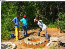
Figure. Digging inside the built beam or collar.
