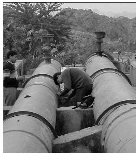
The pipe surface is prepared before the flow meter is mounted
