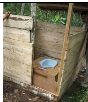
Fig. 13 First stage toilet
