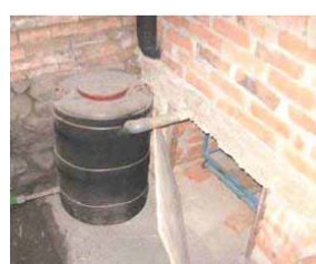
Fig. 16 Single Vault Moveable Container (Indoor dry toilet)
