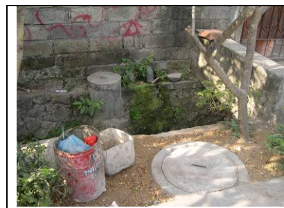
Fig 6 Grease trap and baffle reactor
