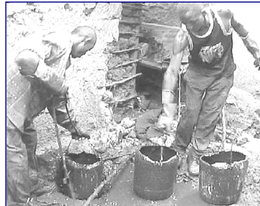
Manual pit emptier at work in a Nairobi slum © Sabine Bongji / WSP
