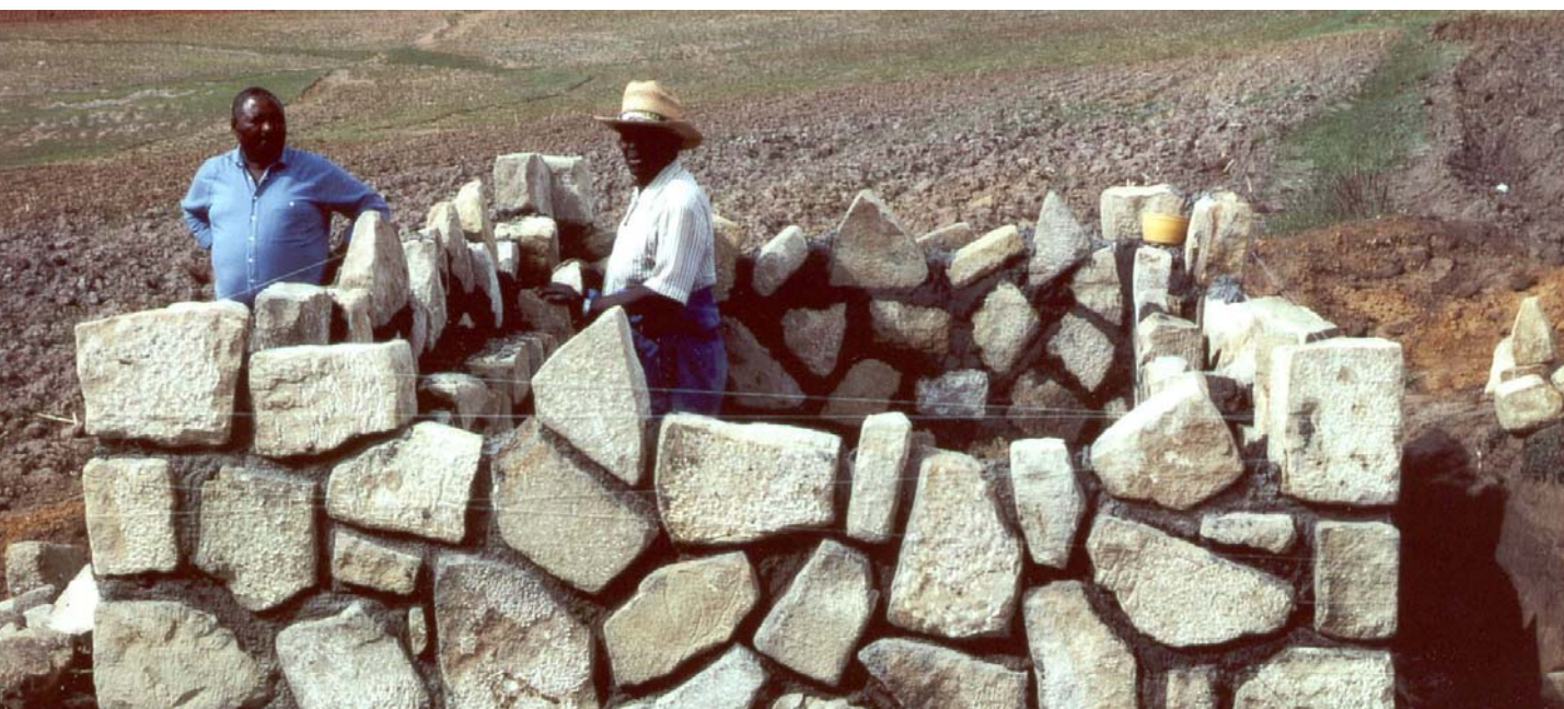
Construction of a reservoir
