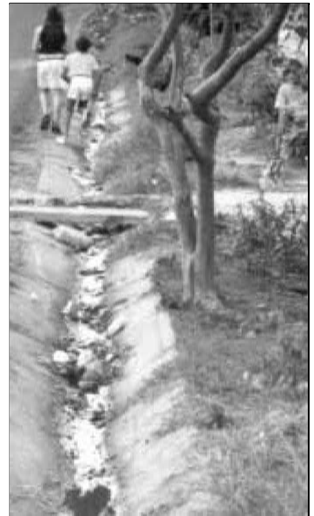
Sewage flowing from a household septic tank into an open canal in Panama
