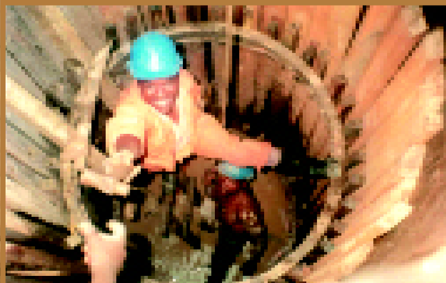
A hand-dug well under construction using temporary caissoning.
