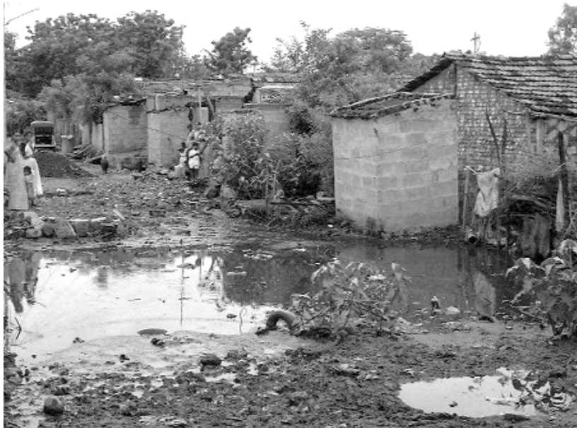
Photo 2: Poor drainage of wastewater in Andhra Pradesh, India
