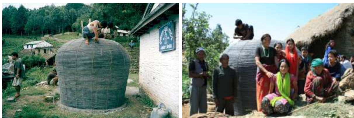
Rainwater harvesting tanks under construction in Nepal
