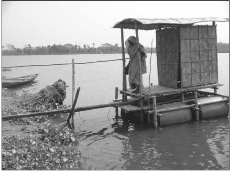
The floating latrine may be used where there is no space on dry land to build a toilet
