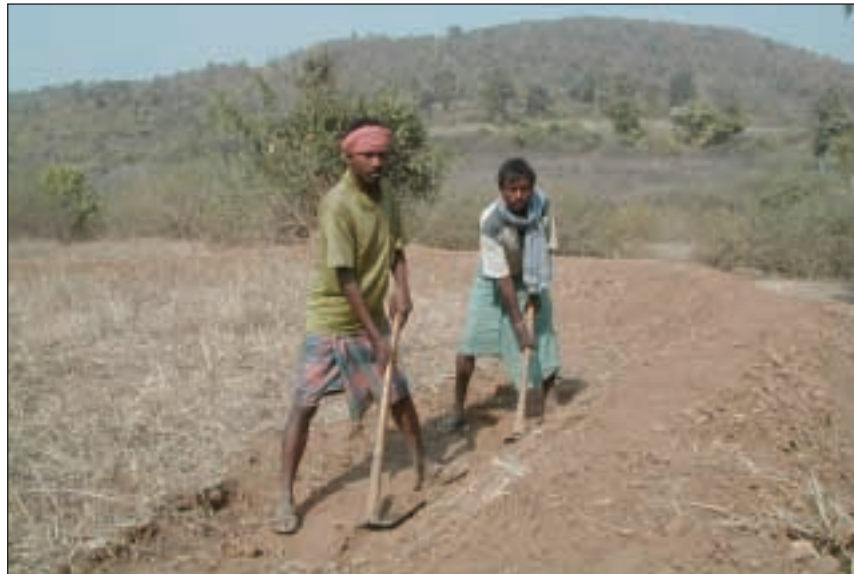
Plate 7) Constructing field bunds to slow rainwater run-off in Bihar, east India. © John Sanchez
