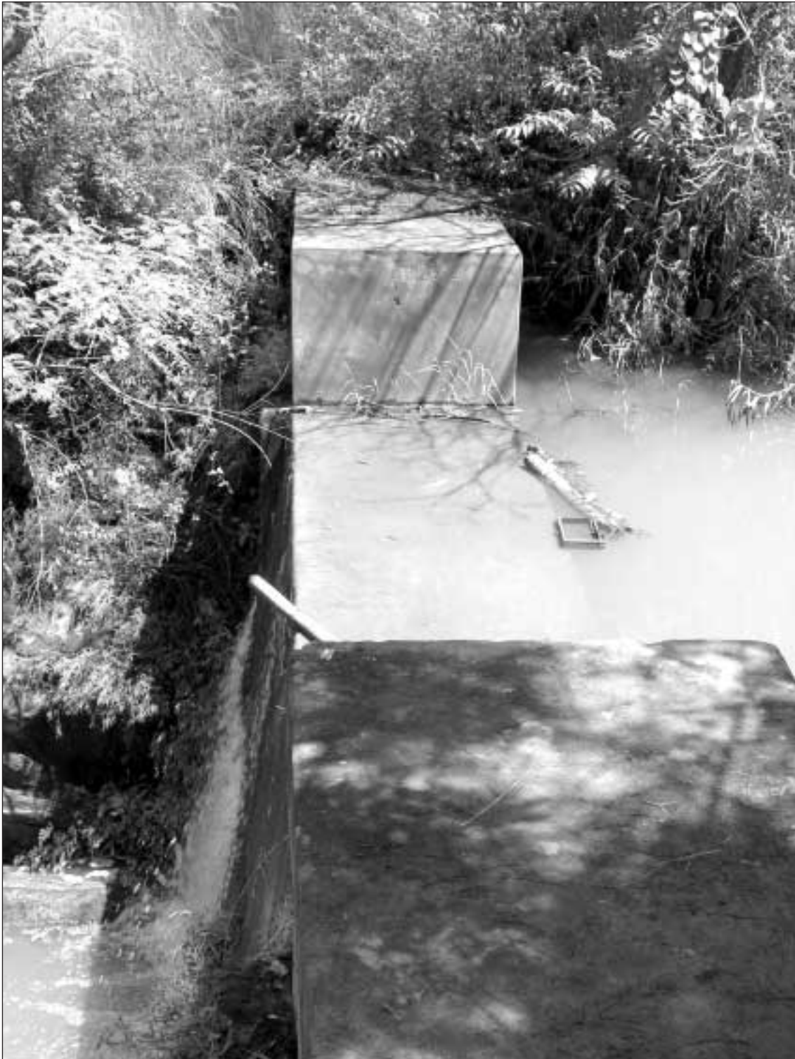
A check dam in the Chabutra Nala watershed, India. © Achraj Bhandari
