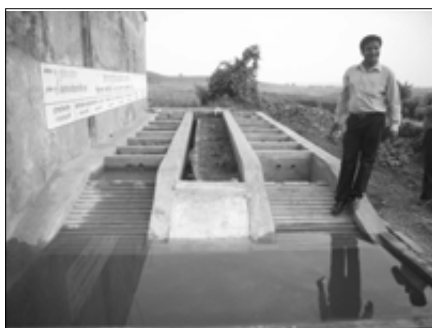
The greywater reuse system in operation
