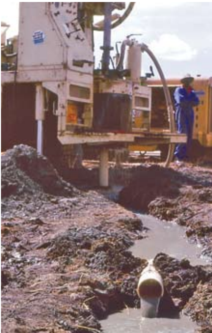
Assessing borehole yield by air-lift testing
