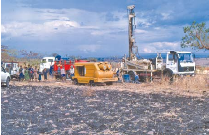
Ready to start drilling in northern Ethiopia
