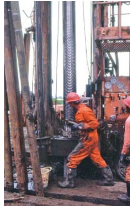
Installation of a steel wellscreen
