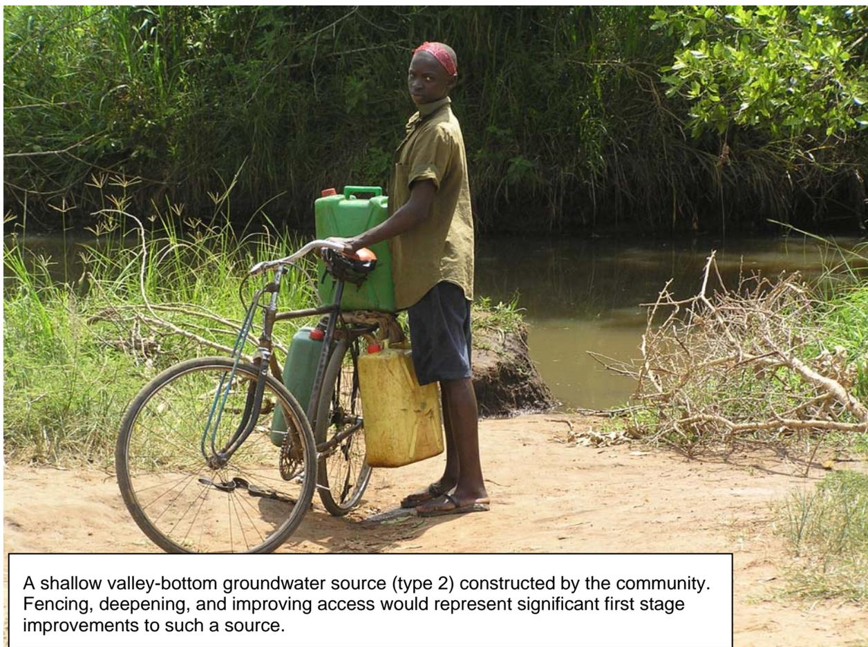
A shallow valley-bottom groundwater source (type 2) constructed by the community. Fencing, deepening, and improving access would represent significant first stage improvements to such a source.
