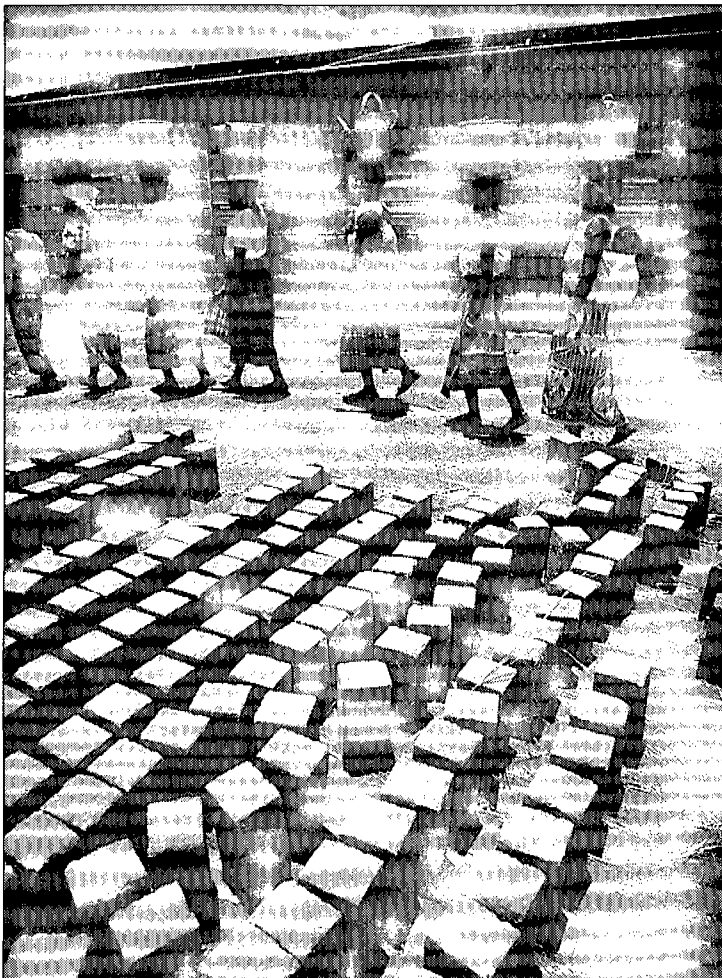
Women are employed in skilled jobs too, particularly block-laying.
