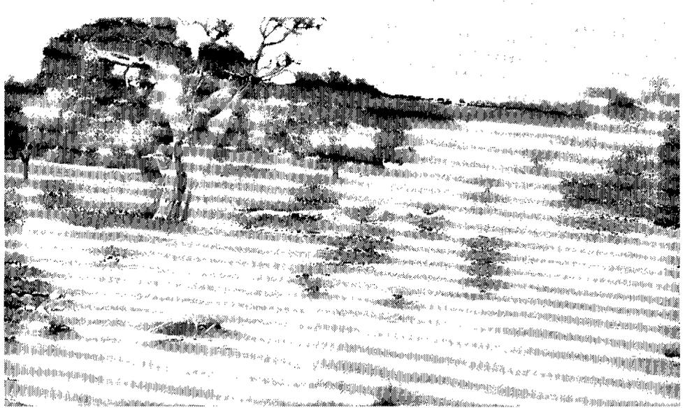
A permeable stone dam built across a gully, with millet cultivated on the sediment trapped upstream.
