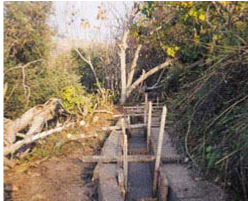
Photo courtesy of the WEPIA Program The canals in this photo were lined with cement to decrease percolation of water into the soil.
