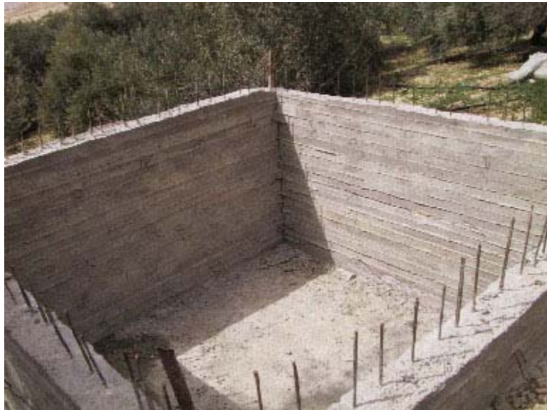
Photo courtesy of the WEPIA Program In the Al-Eina Valley, farmers depend on natural springs for irrigation. Reservoirs, as shown in the photo, were built to store water to allow farmers to irrigate their crops more regularly.
