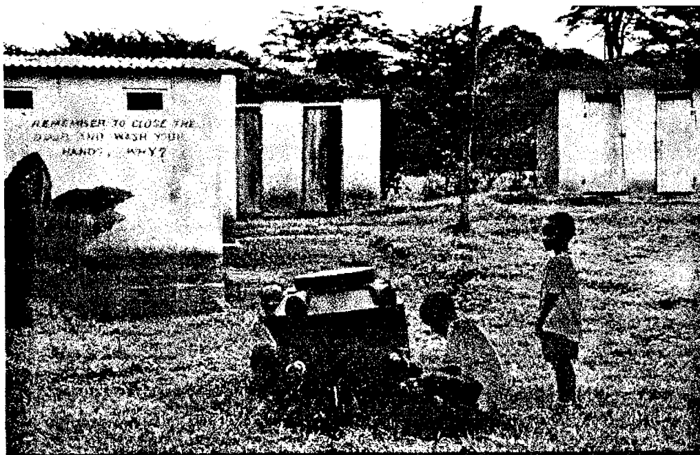
Picture 7: One example of educational message on the latrines wall.
