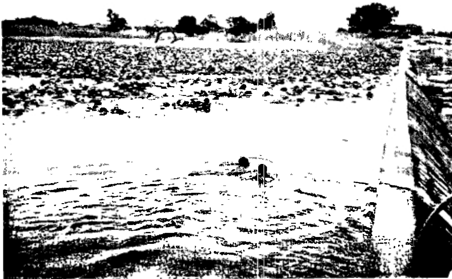
Photo 3 Kori-kori dam, built in 1973, is 2 meters high and 234 meters long Besides irrigation and livestock watering, the reservoirs are used for bathing, swimming, domestic uses, fishing, and sometimes drinking The reservoirs typically contain large quantities of aquatic vegetation which provide a habitat for the snails which transmit schistosomiasis Also apparent in this picture is leakage at the dam's downstream base
