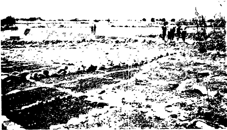
Photo 2 Dourou dam built in 1984, 3 5 meters high and 131 meters long Villagers bring the soil to garden plots adjacent to the dam and build up gardens on top of the rock
