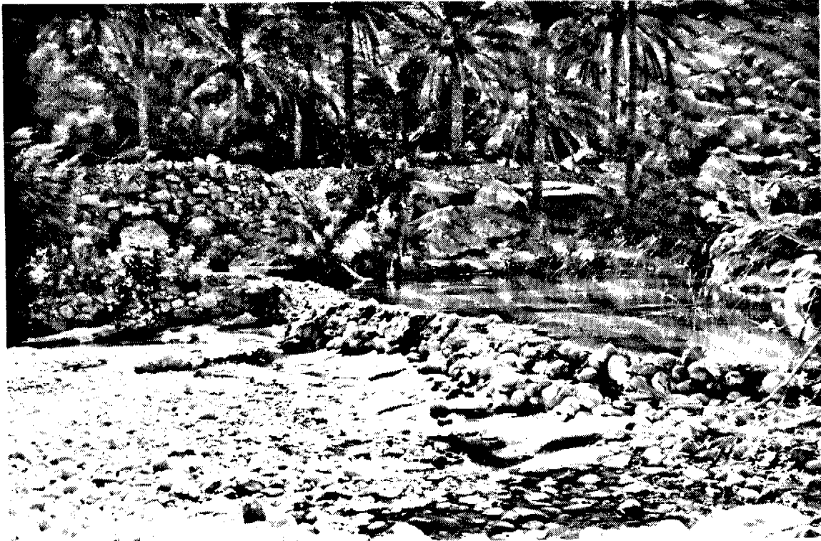
A typical Ghayl Falaj Intake Structure at Mugal
