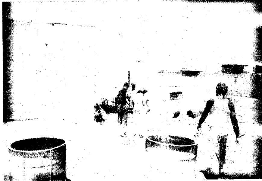
Manhole shutterings are being prepared during laying of lane sewers in Gulshan-c-Zia.
