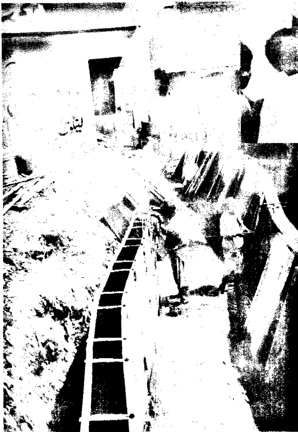
'L' Block nala: Defective work, faults in alignment and levels - needs constant rectification.
