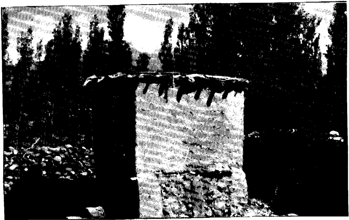
Figure 1. Outside and inside views of the experimental twin pit compost latrine
