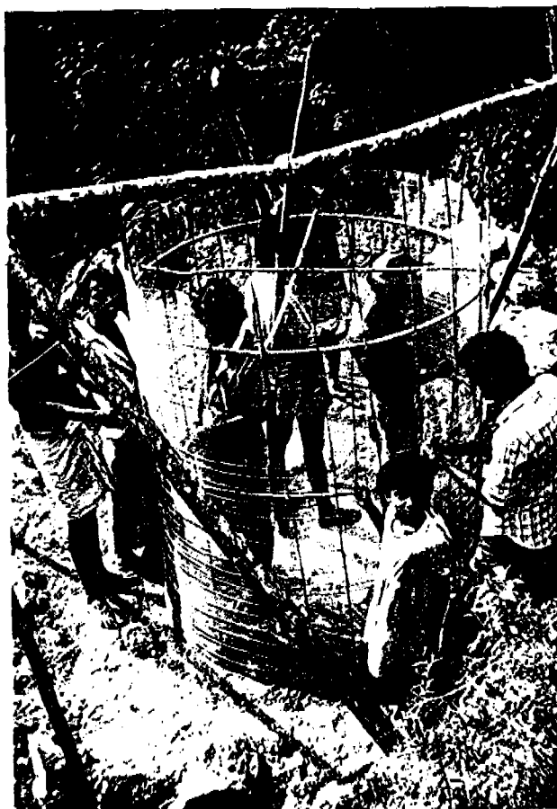
Photograph 4: Technicians and villagers together Constructing a ferro cement tank (Arthacharya)
