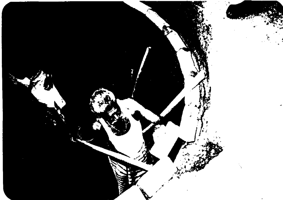
Photograph 3: Villagers Building a least-cost rain water Storage Tank (Hapugoda)
