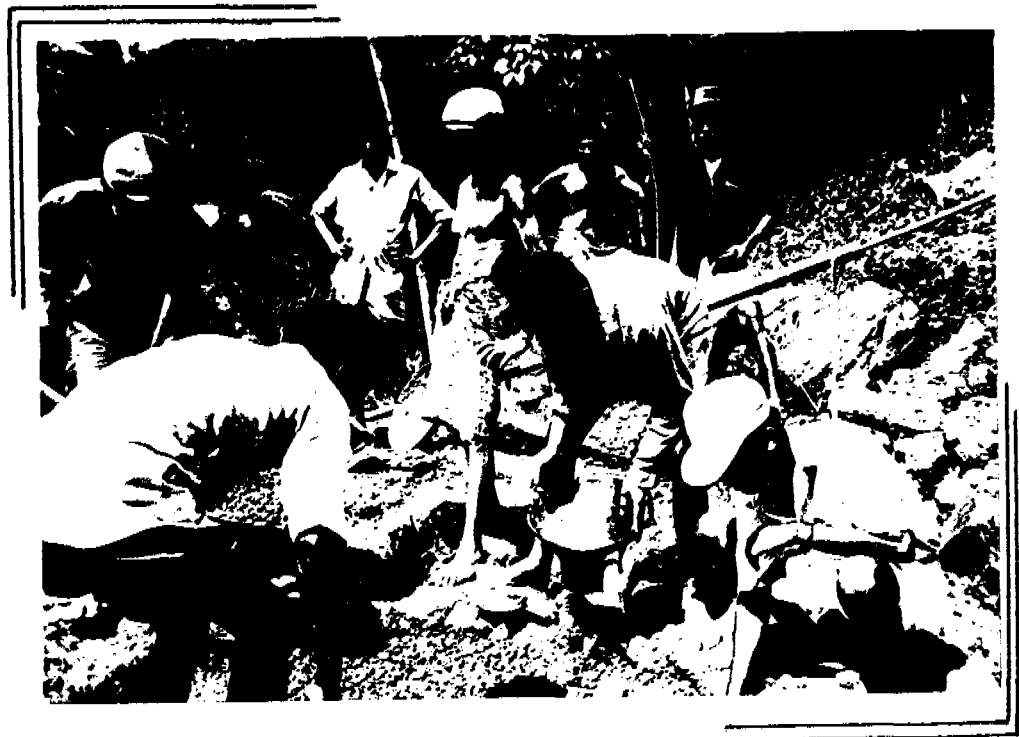
Photograph 1. Preparing the Foundation for the Storage Reservoir (Arthacharya)
