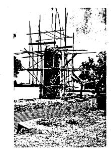
Fig. 4. Brickwork tower encased in ferrocement.
