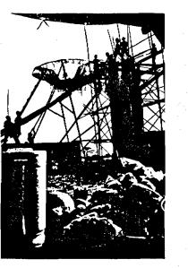
Fig. 6. Tank bottom reinforcement cage lifted manually.
