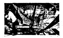
Fig. 5. Saucer shaped bottom of tank.
