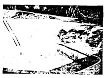
Fig. 6. Plastering the slopes with ferrocement.
