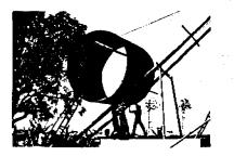
Fig. 7. Formwork of tank rolled up to position.
