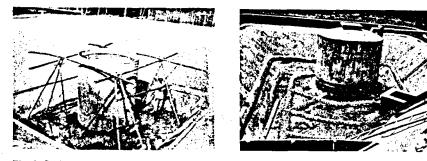
Fig. 8. Setting up of the mould for the collection well,
