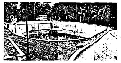
Fig. 2. The slow sand filter. The collection well is seen in the middle and the pole valve is on the right,
