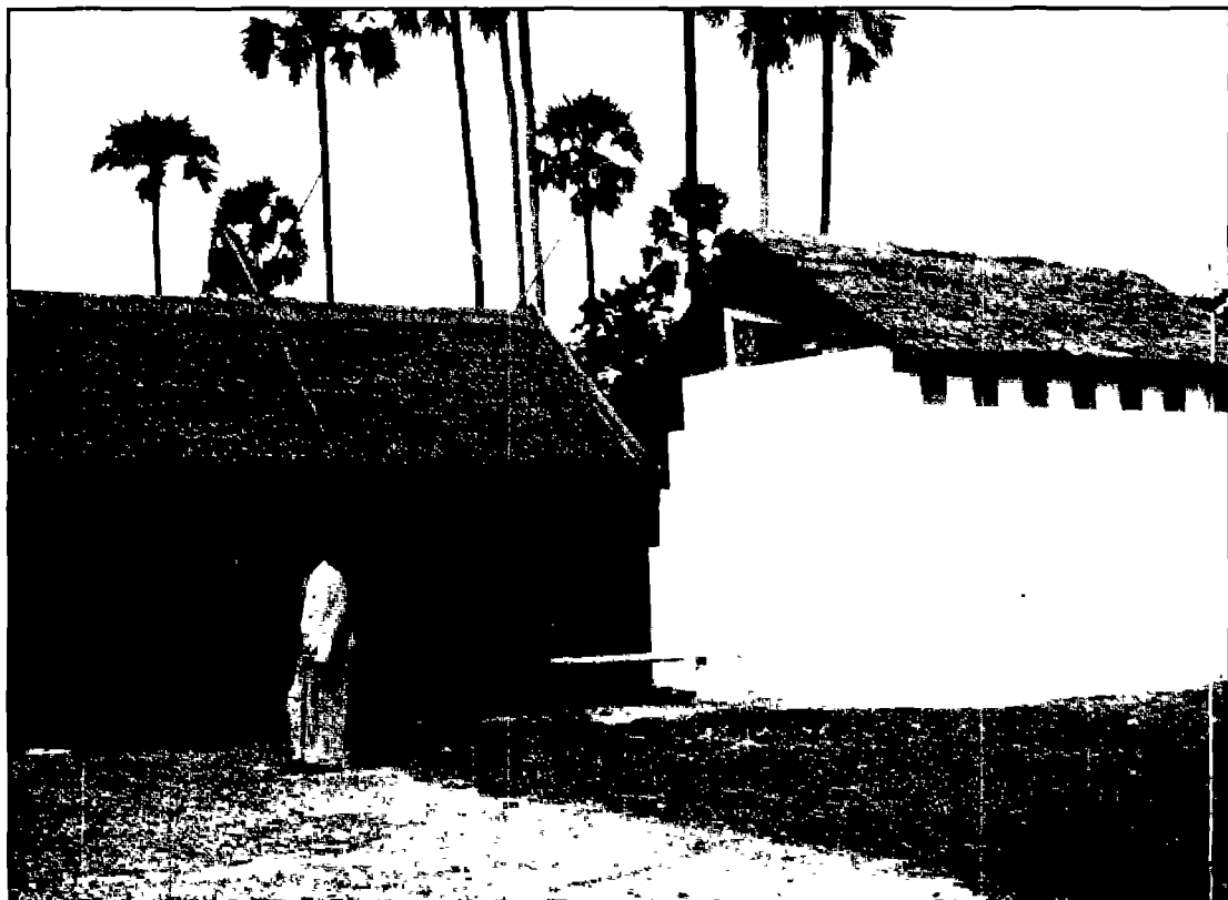
A newly completed pumphouse, with its concrete water storage tank on the right
