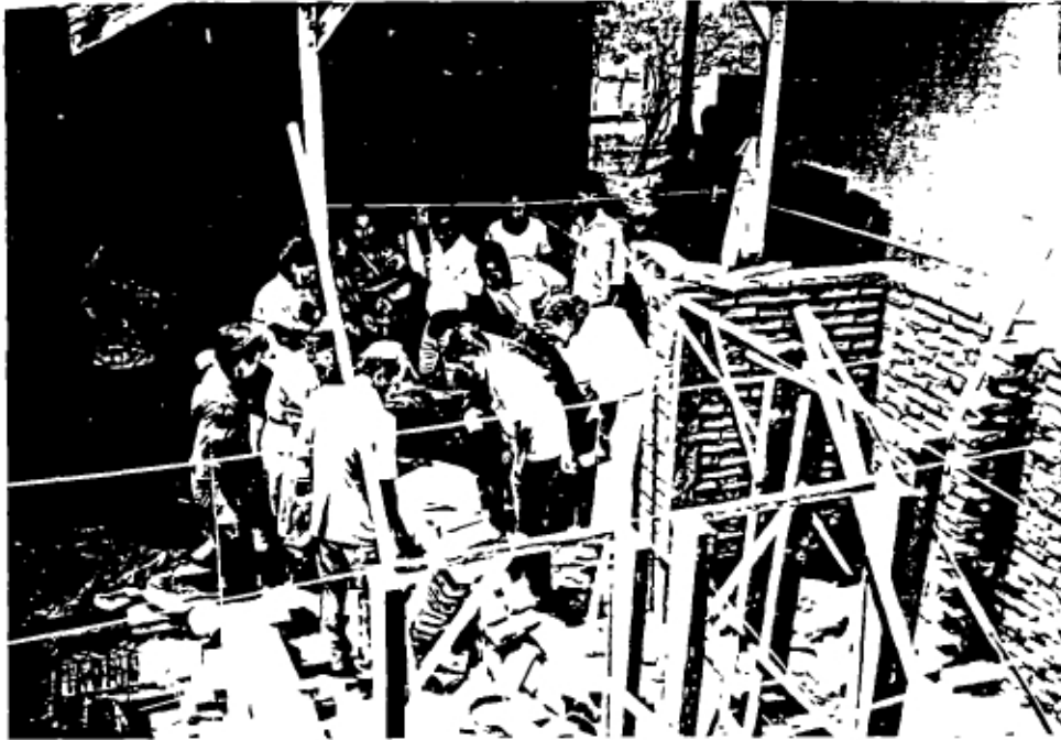
parents visiting construction site
