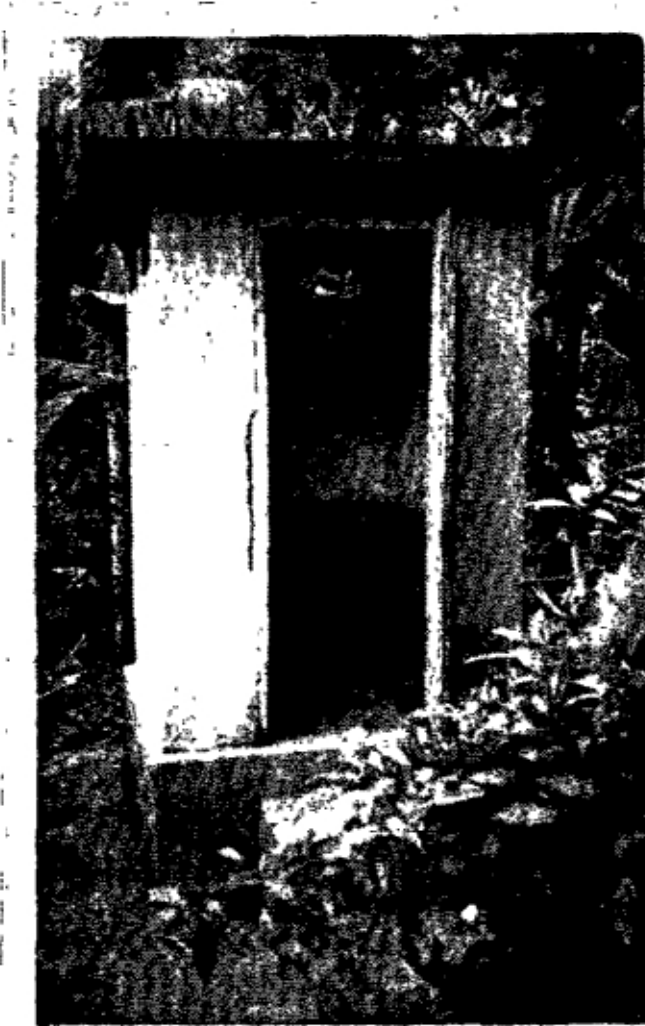
Fig. 6-2. Pit latrine with concrete slab, brick walls and concrete roof, and water connection inside the toilet. Not common in the village
