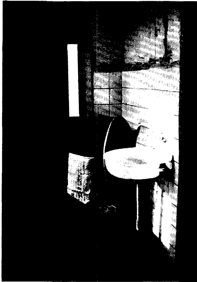
Photo 28: First floor restroom, Tbilisi Hotel, Kutaisi
