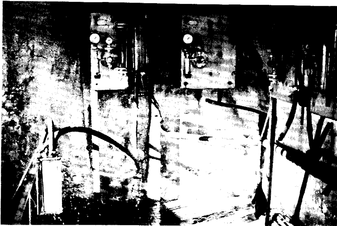
Photo 14: Chlorinator—beyond repair
