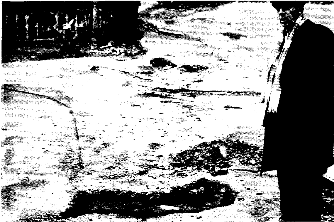
Photo 5: Water leak/broken line in street
