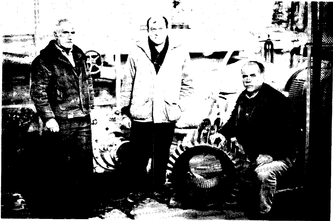
Photo 9: Example of motor destroyed by "off-frequency" operation—Kutaisi Water System
