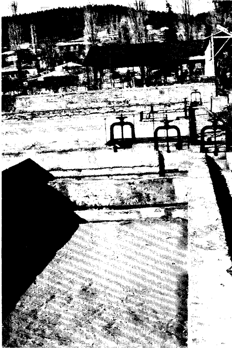
Photo 17: Filter beds in poor condition
