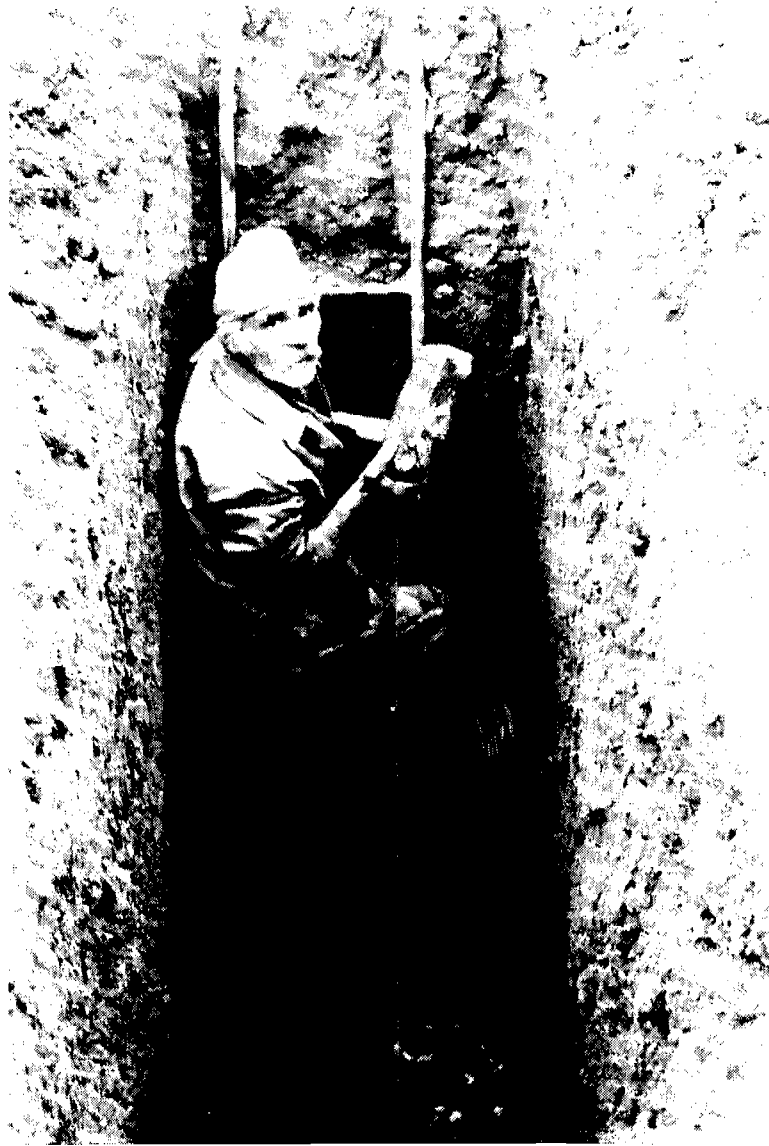
Photo 22: Unplugging sewer (c)
