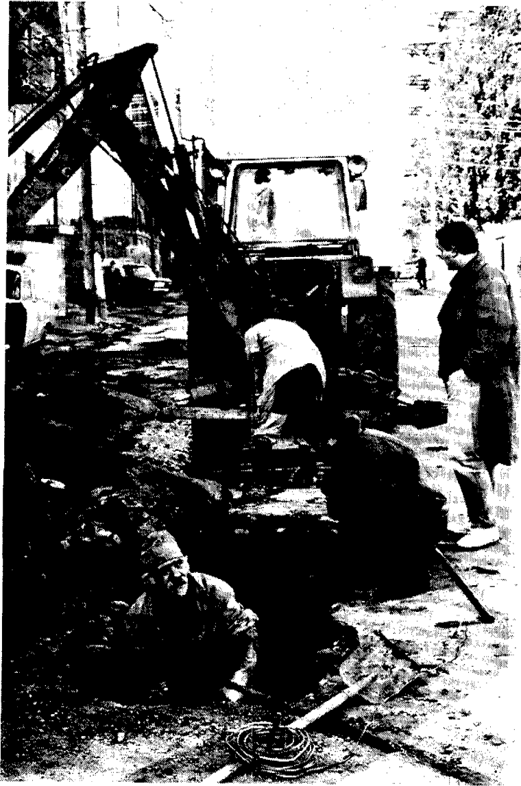
Photo 20: Unplugging sewer (a)
