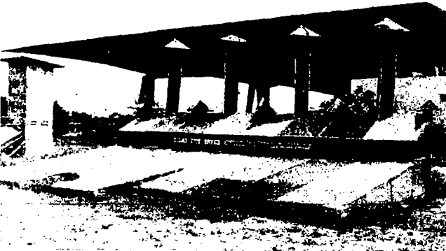
Solar rice dryer built at AIT.
