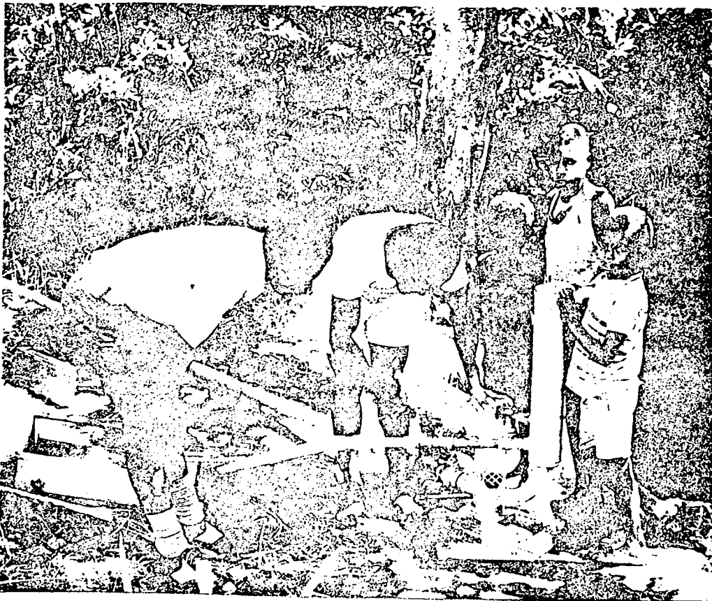
FIG. 4 The hydraulic ram at the Waritzian Community School being repaired by one of the school teachers and a technician from the University of Technology.
